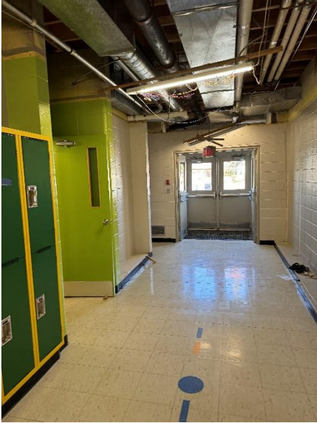
Northwest Hallway / Asbestos Vinyl Floor Tile (speckled beige)
