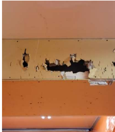
Interior Fixed Partitions
