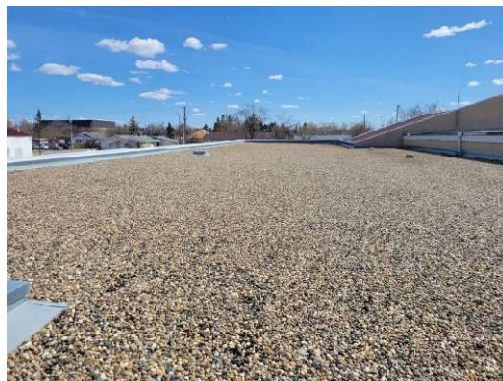
Built-up Bituminous Roofing (Asphalt & Gravel)
