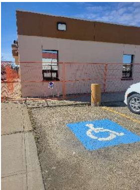
Parking Lot Signs
