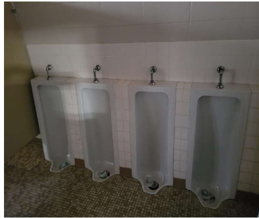
Tile Wall Finishes
