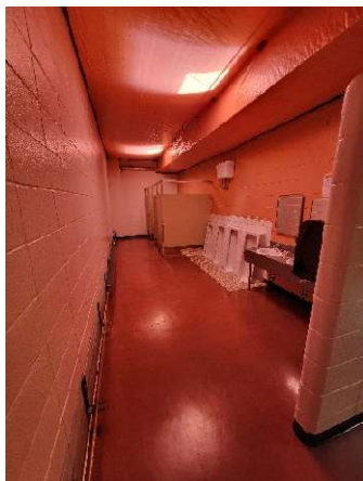
Fabricated Compartments (Toilets/Showers)
