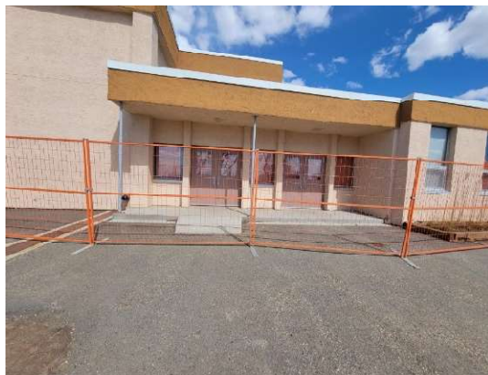
Exterior Utility Doors
