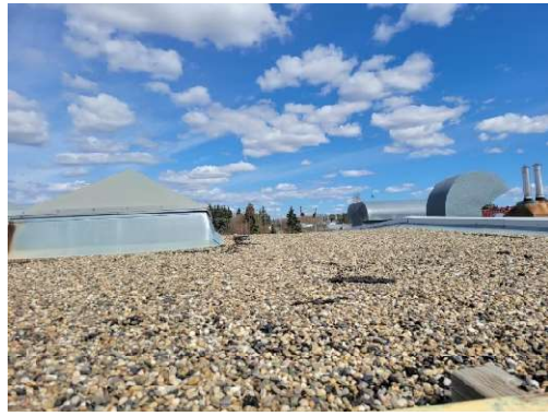
Built-up Bituminous Roofing (Asphalt & Gravel)
