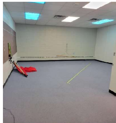
Interior Wall Painting
