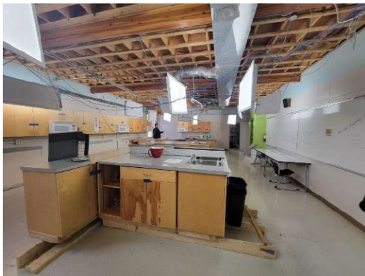
Typical 1962 & 1967 wood structure.
