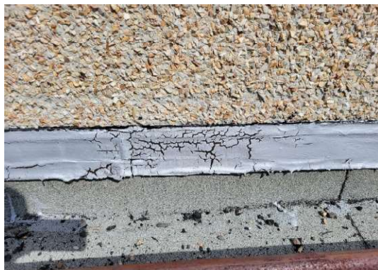
Built-up Bituminous Roofing (Asphalt & Gravel)
