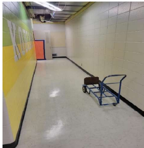
Interior Fixed Partitions
