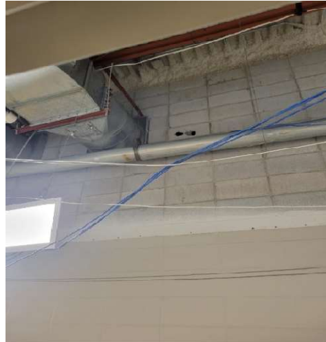
Interior Partition Firestopping
