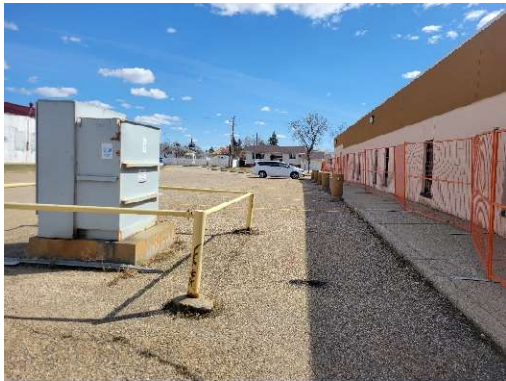
Rigid Pedestrian Pavement (Concrete)
