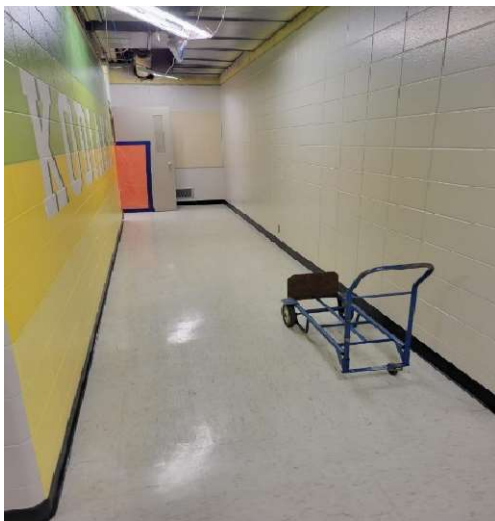
Interior Fixed Partitions
