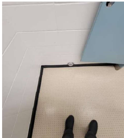
Interior Fixed Partitions
