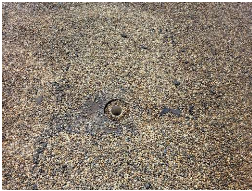
Built-up Bituminous Roofing (Asphalt & Gravel)
