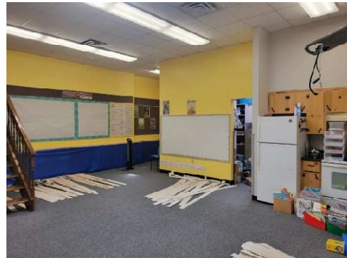
Interior Wall Painting
