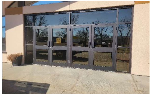
Rigid Pedestrian Pavement (Concrete)
