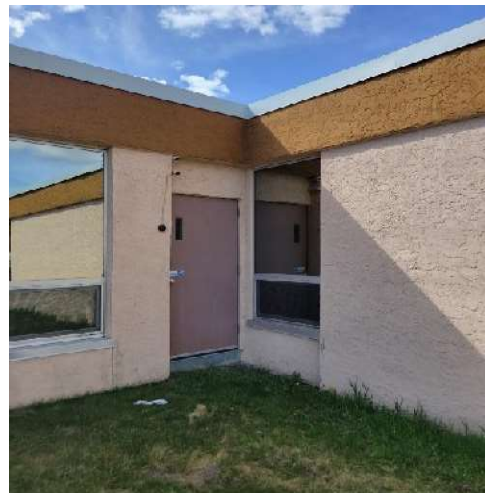
Exterior Utility Doors
