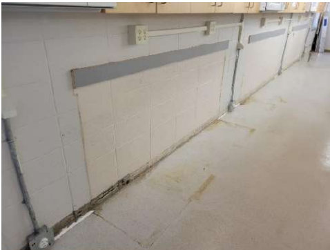
Interior Wall Painting
