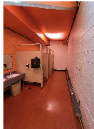
Fabricated Compartments (Toilets/Showers)
