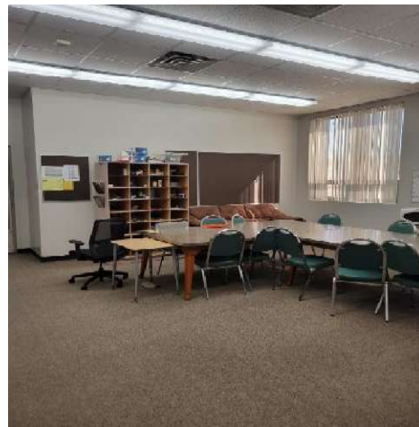
Acoustic Ceiling Treatment (Susp. T-Bar)
