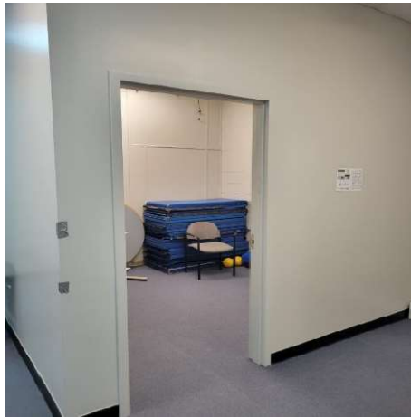
Interior Fixed Partitions
