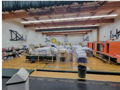
Gym glulam structure
